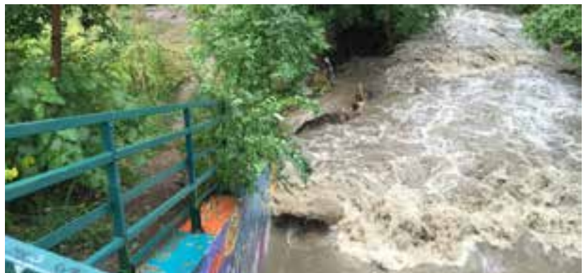
The channel, surrounded by impervious land cover, can flood quickly from a rain event, as evidenced by recent rains in 2016.
