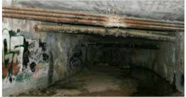
Utilities passing through structure at Cache la Poudre Street.
