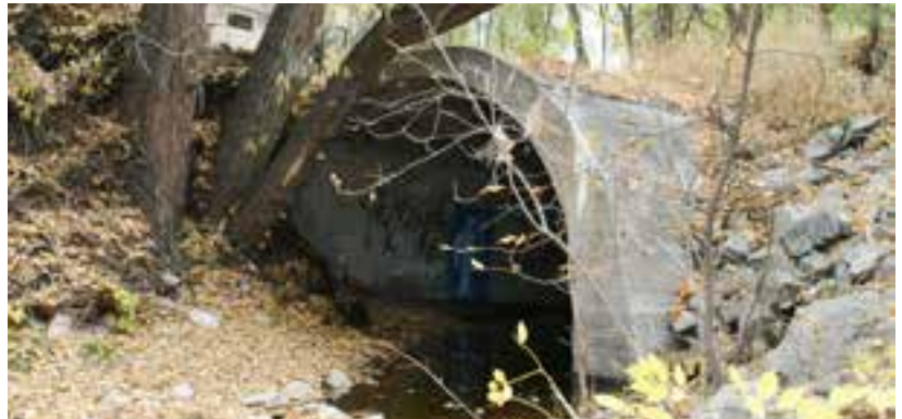
One-hundred year old culvert structure at Cache la Poudre Street.
