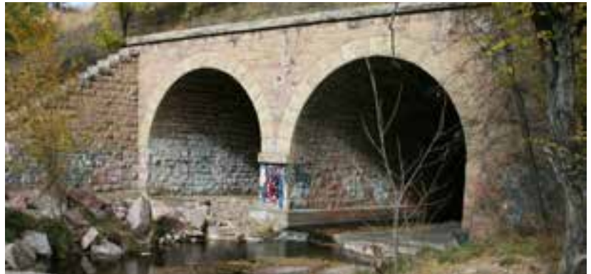
The historic railroad bridge located to the south of Fountain Boulevard was an important part of the historic transportation infrastructure.
