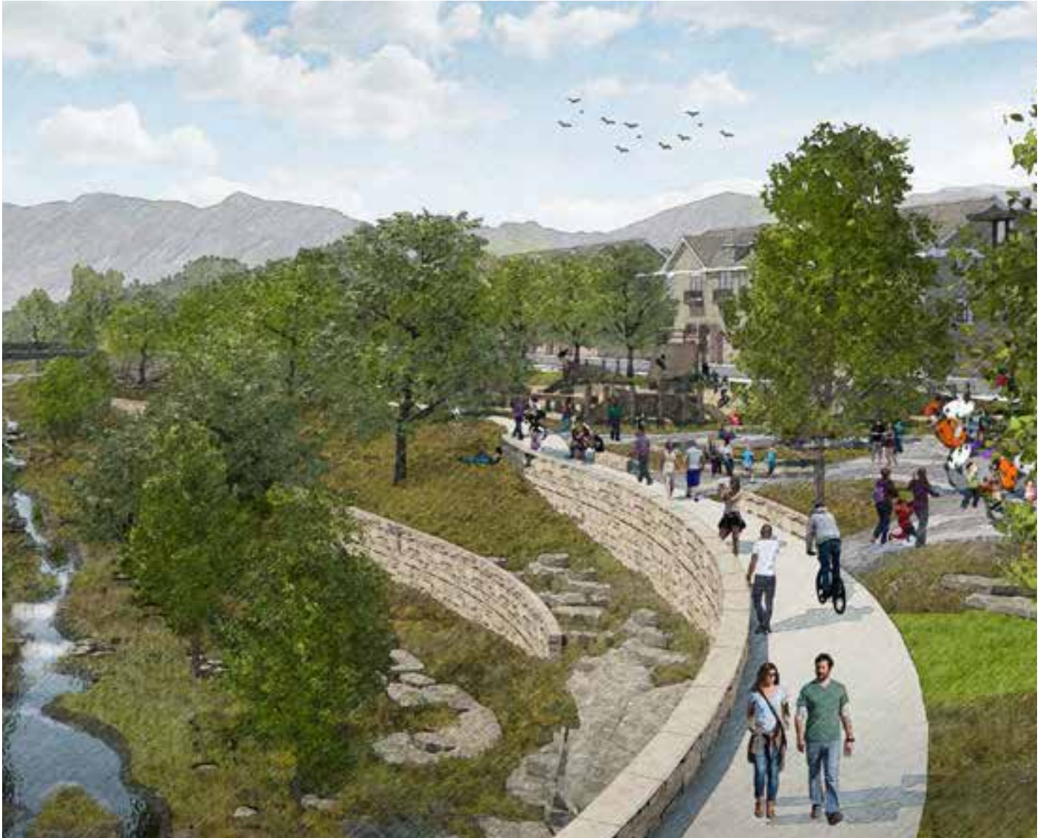
The narrow channel is replaced with new side-slope, channel elevation and the introduction of meanders along with usable parkland and an urban park with programs and recreation that enhance the redevelopment potential along Wahsatch Avenue.
