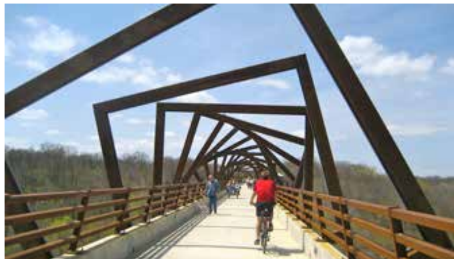
This example is similar to the proposed bridge for Rio Grande Street, which would allow crossing at street level for pedestrians and bicyclists.
