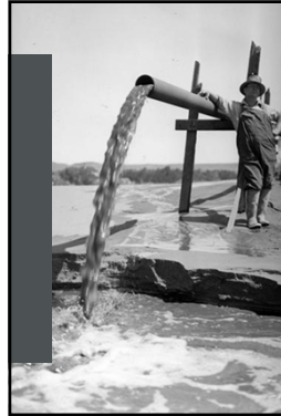
Photo: George Hager stands near a pipe that drains the sand, water, and tailings mixture from the Golden Cycle Mill in El Paso County. Source: The Gazette
