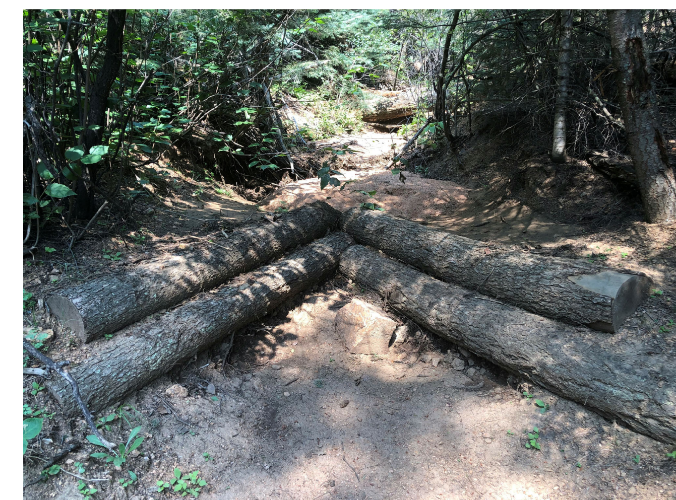
7 Timber Cross Vein Example - Look uphill from trail tread 10 Not To Scale
