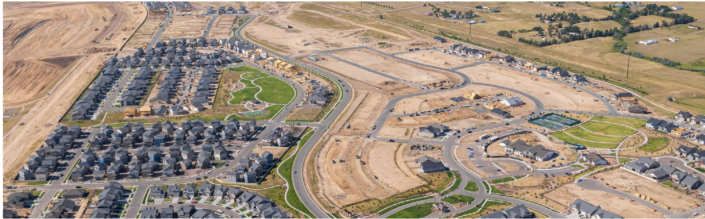
Banning Lewis Ranch development and construction
