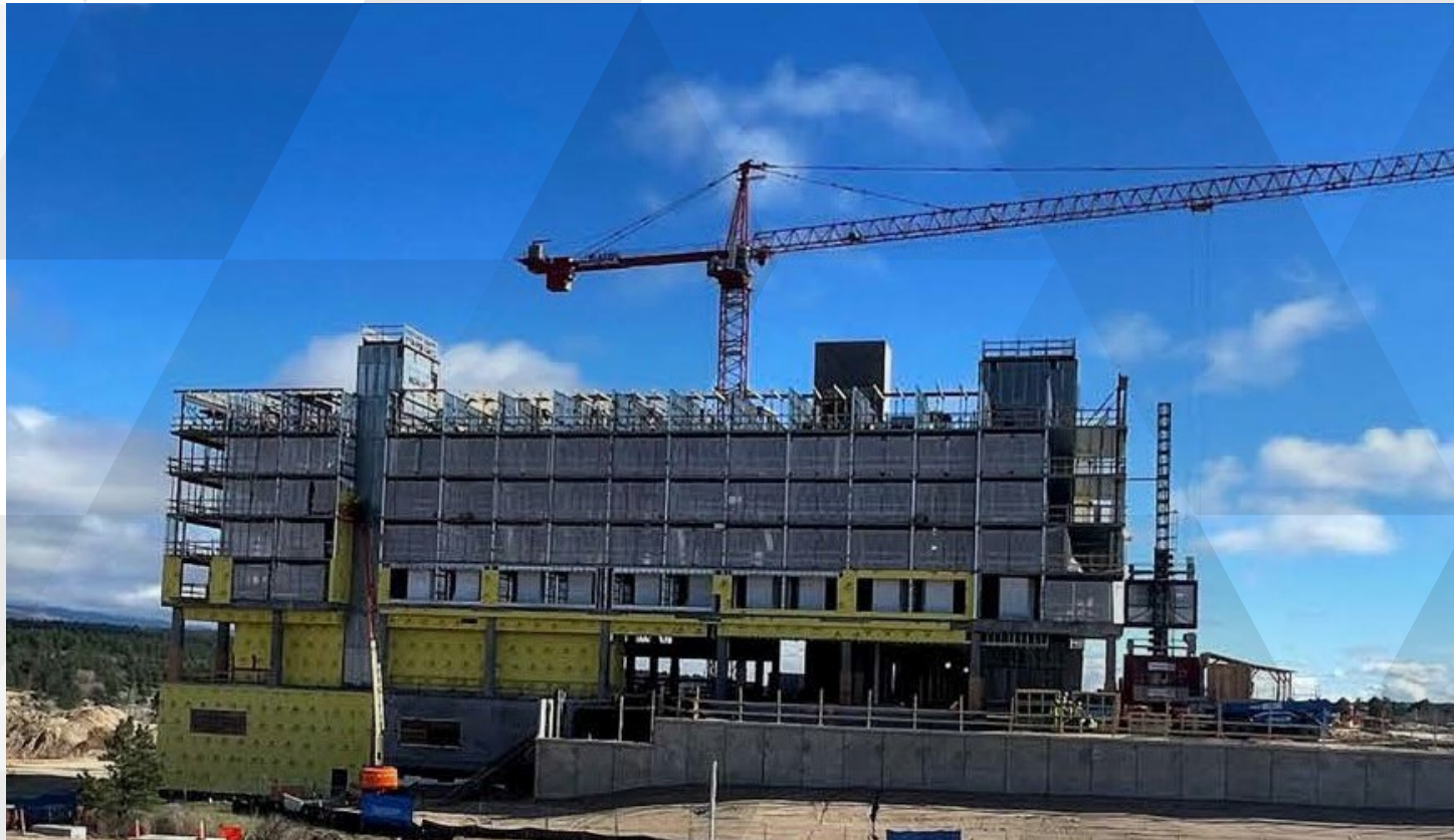
United States Air Force Academy Hotel under construction
